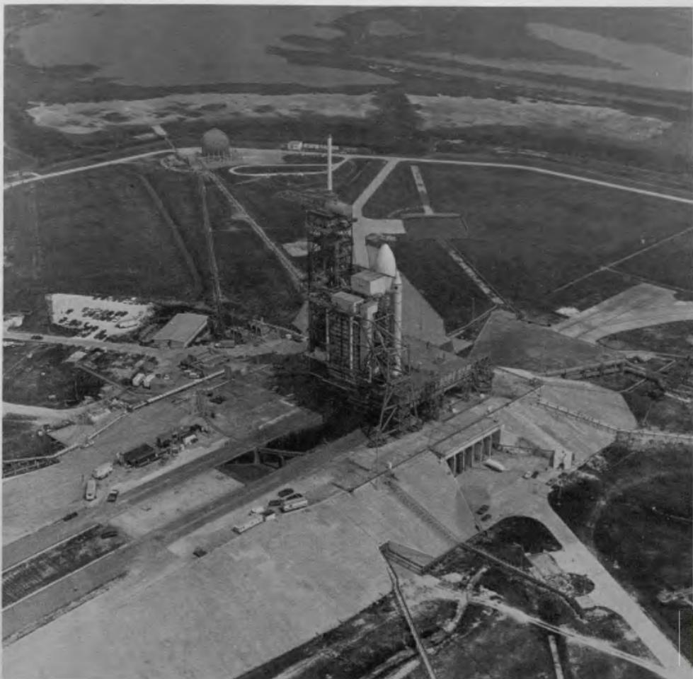
Figure 18. Rotating Service Structure in Access Position.
